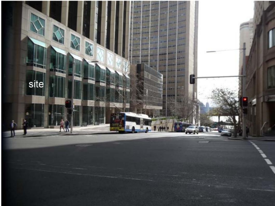
Figure 16: Existing eastern elevation viewed from the corner of Bridge and Phillip Streets
