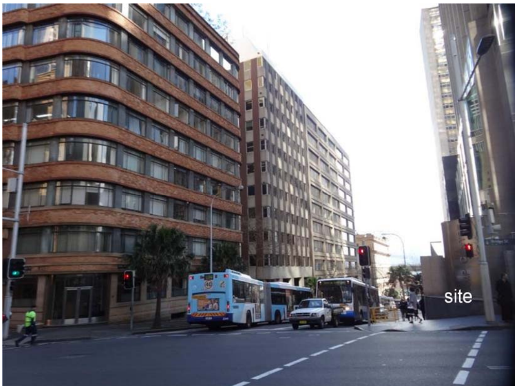
Figure 5: Adjacent buildings located on the western side of Young Street, view looking north
