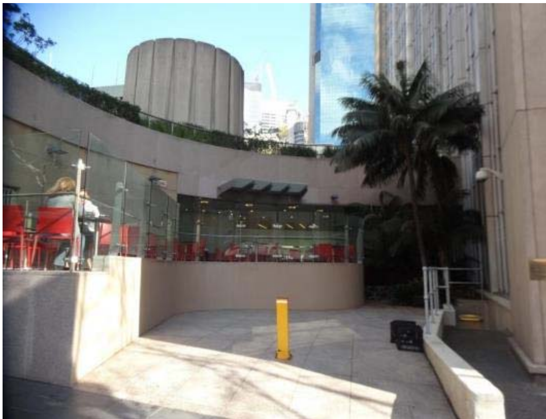
Figure 13: View west towards interface with 33 Alfred Street building from Phillip Street
