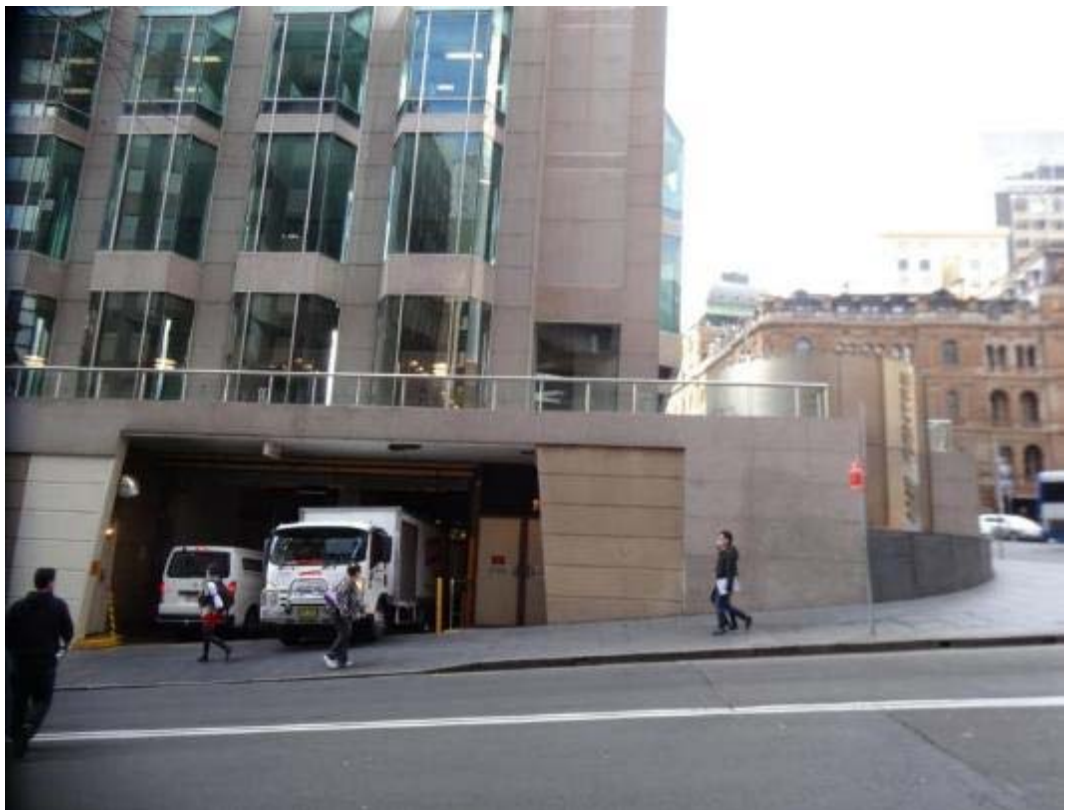
Figure 7: Existing AMP tower loading dock, corner Young and Bridge Streets
